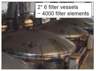
By cooling the gas to 400°C, impurities in the fuel, such as alkali chlorides, Pb and Zn, turn to solid form and are more easily removed. The gas impurities are removed inside 12 cooling chambers containing 300 high temperature ceramic candle filters, each collecting unwanted particles while allowing the gas to pass through. A nitrogen pulse every minute ejects collected dust, which falls to the chamber floor for removal.
